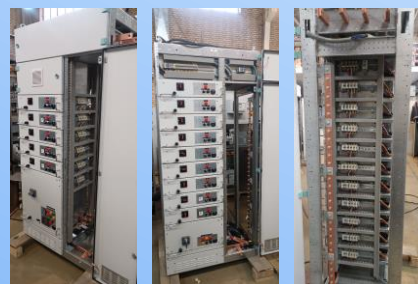
Withdrawable Panel (Sivacon)
